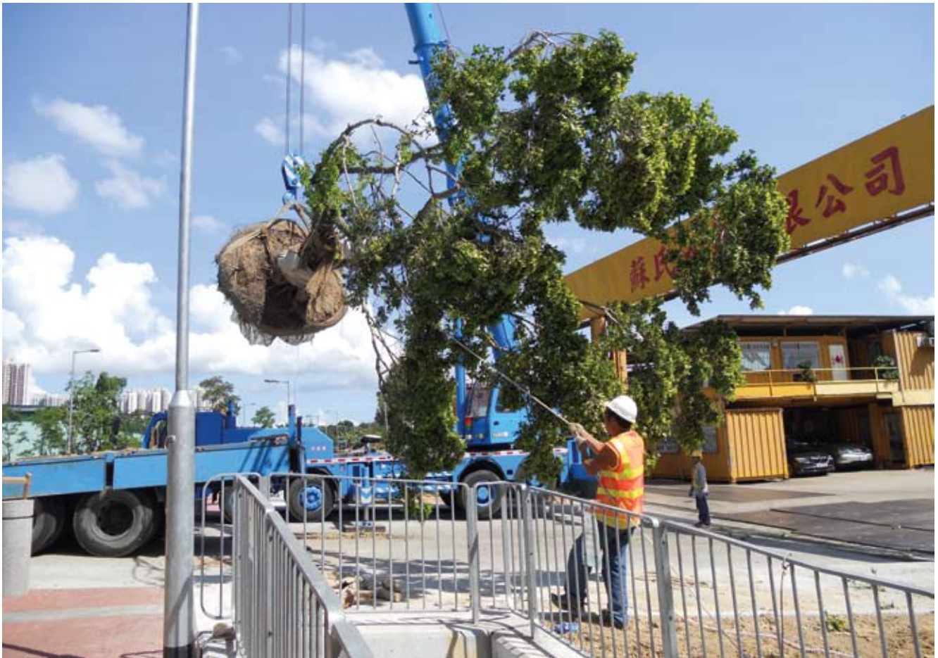
Photo 4: Lifting and handling mature street trees
