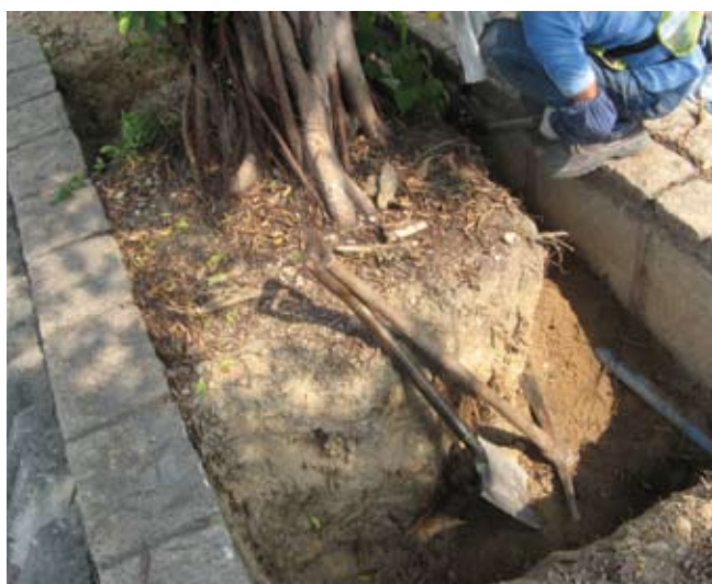
Photo 2: Excavating trees from roadside locations in Hong Kong
