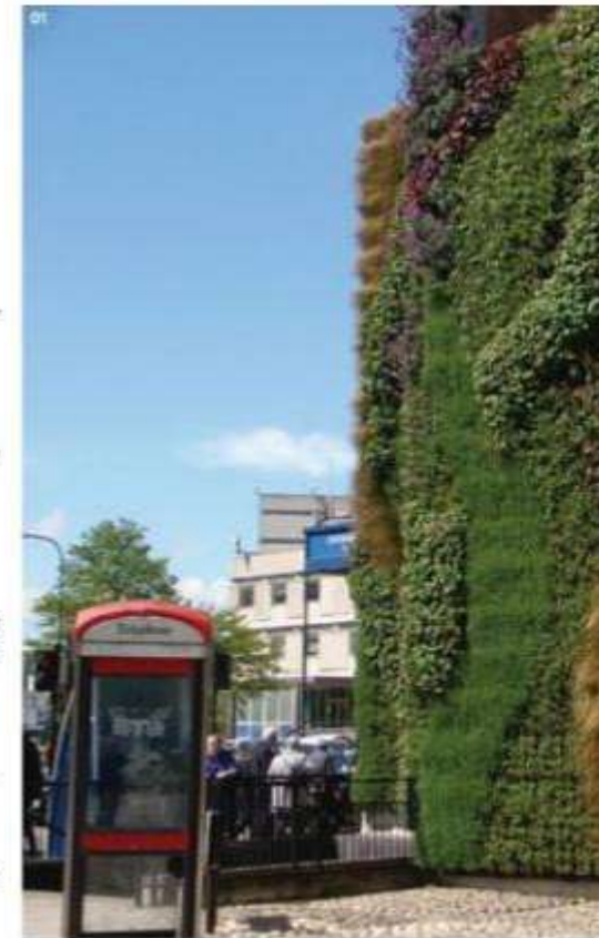
01 Edgware Road green wall, London, Transport for London
