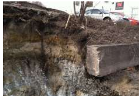
Rooting soil under parking lot
