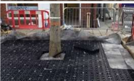
Arbor Raft (Hybrid system – depends on compacted sand below raft for soil volume)
