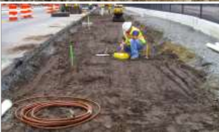
Compacted Sand Structural Soil
