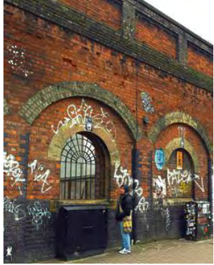
Sclater Street Boundary Wall
