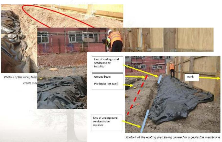
Note the location for the ground beam (600mm deep)
