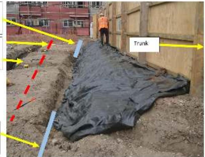
Photo 4 of the rooting area being covered in a geotextile membrane
